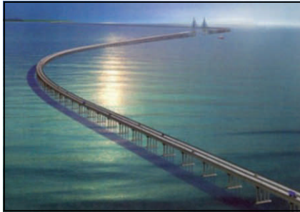
Lake Pontchartrain Causeway Bridge
