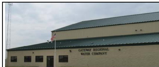
CDAP funds helped build the Gateway Regional Water Company which was designed by Heneghan and Associates.
