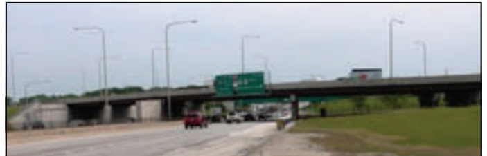
Mannheim Road over the I-190—one of Thompson’s biggest design jobs in the Chicago area.
