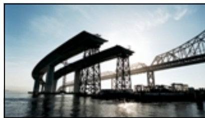
San Francisco -Oakland Bay Bridge
