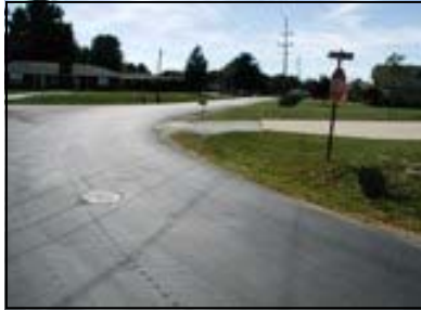
Fairgrounds Avenue—In Progress City of Jerseyville
